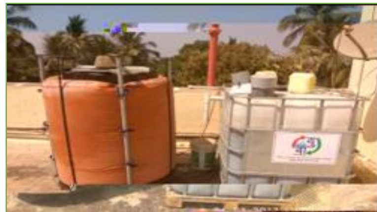
Biogas Plant Installed
