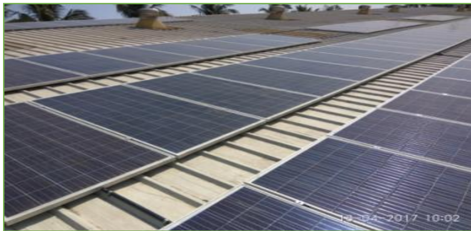
Solar Panel Installed on the roof top
